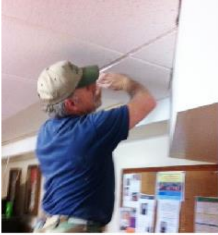
John Seay installs a ceiling panel.
