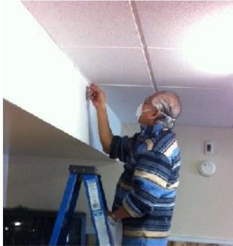
Rudy Nartea installs caulking around the panel edges.
