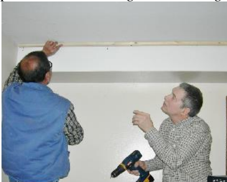
Quintin Mugas and Bob Lundberg install grids on ceiling.
